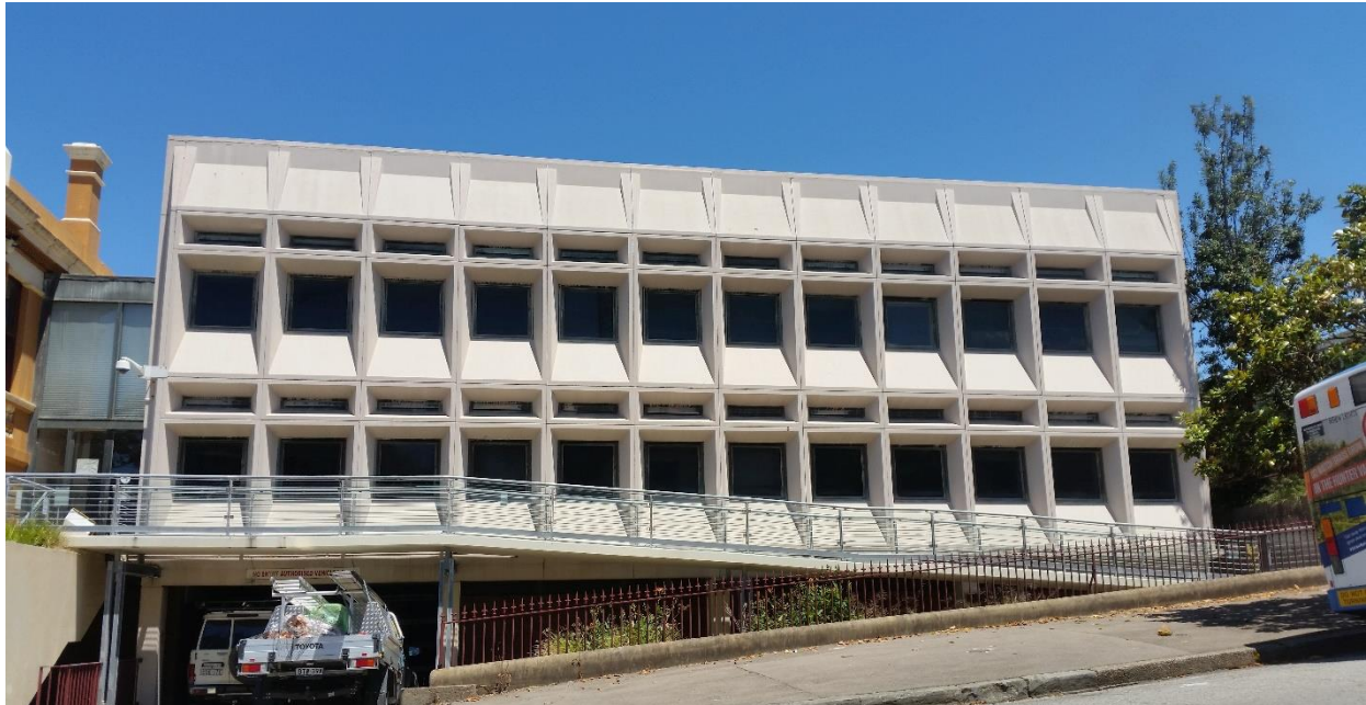
Figure 18: Existing Supreme Court Building and access ramps fronting Church Street (photo looking south)
