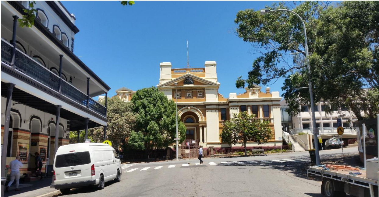
Figure 17: Existing former Courthouse building fronting Church Street opposite intersection with Bolton Street (photo looking south)
