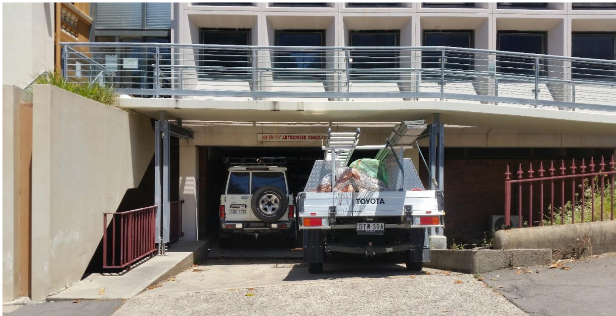
Figure 19: Existing 2-way driveway from Church Street to Supreme Court Building car park (photo looking south)
