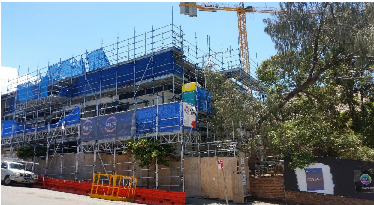
Figure 5: New 5-storey 'Parque Apartments' currently under construction to the north-west of the site (photo looking north-west)
