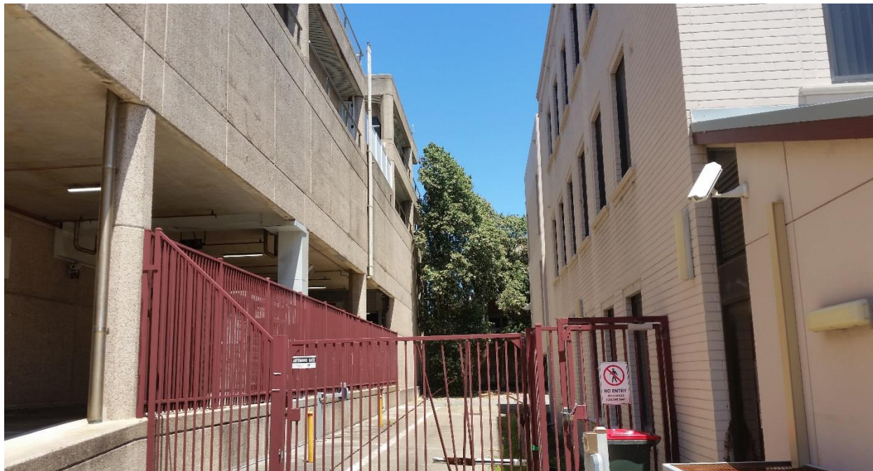
Figure 22: Existing gated service driveway off Church Street along site's eastern boundary, adjoining Newcastle Police Station (looking south)
