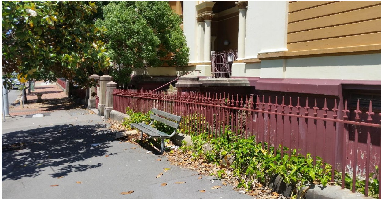
Figure 23: Site frontage to Church Street, including original front fencing and plinth (looking west)
